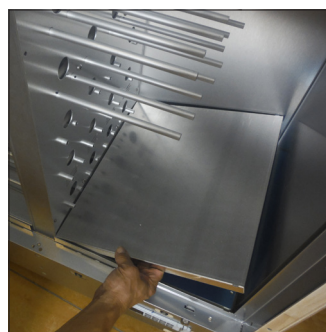
A3. Remove the alluminium panel
