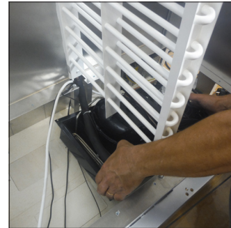
C6. Unscrew the screws holding it and extract the cooling unit
