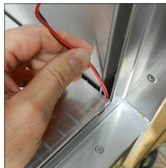
E7. Insert the new LED strips in the aluminium profiles and extract the 4 cables from the holes in the basin
