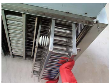
Figure 6-1 take out the EF and air flow divider
