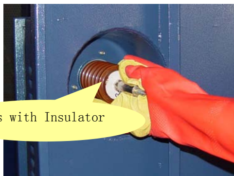
6.2.3 Figure 6-5 Clean Insulator
