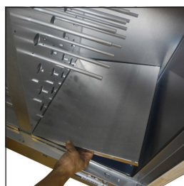
A3 . Remove the aluminium panel
